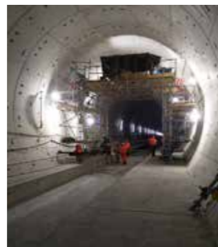
Tunnel tube with mobile scaffolding for manual testing.
